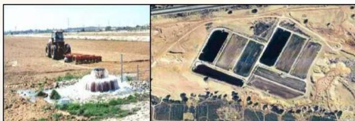
Figure 2 - Soil Aquifer Treatment
