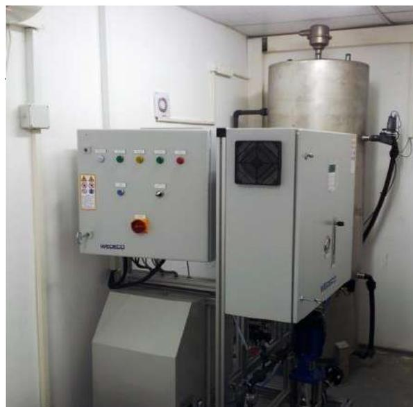
Figure 3 - ozonator at the Shafdan WWTP R&D center
