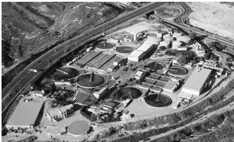
45 Figure 1. “Rincón de León” WWTP-WRP (EPSAR)
