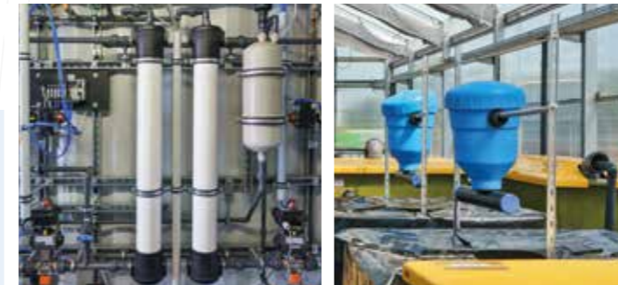
▲ Ultrafiltration (left); automatic feeding system of the aquaponics (right)
