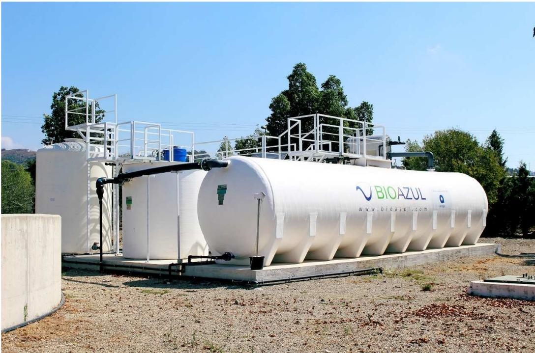
Figure 9: MBR unit of RichWater technology
